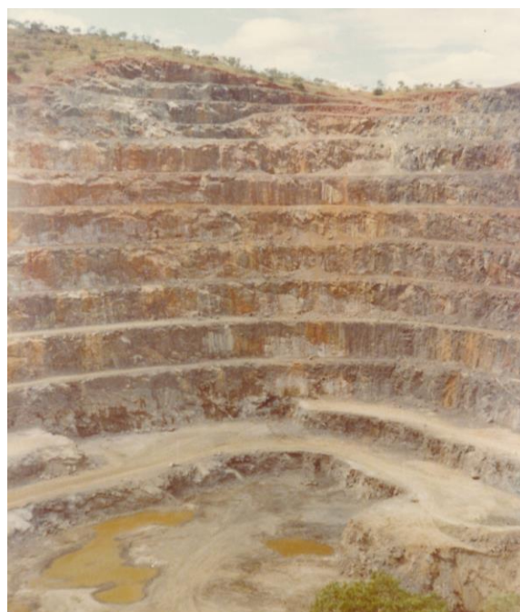
Figure 2 Looking south east – Centre of picture is the first 24m high final batter in Queensland. - 1980
