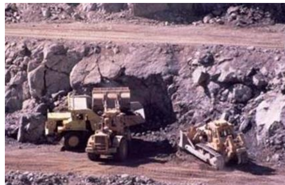
Figure 2 North- South Production Bench showing multiple open joint sets
