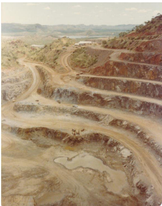
Figure 3 Looking North, Joint sets resulting in production bench crest and wedge failures - 1980
