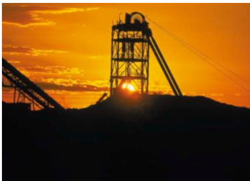
Scuddles Project -Western Australia
